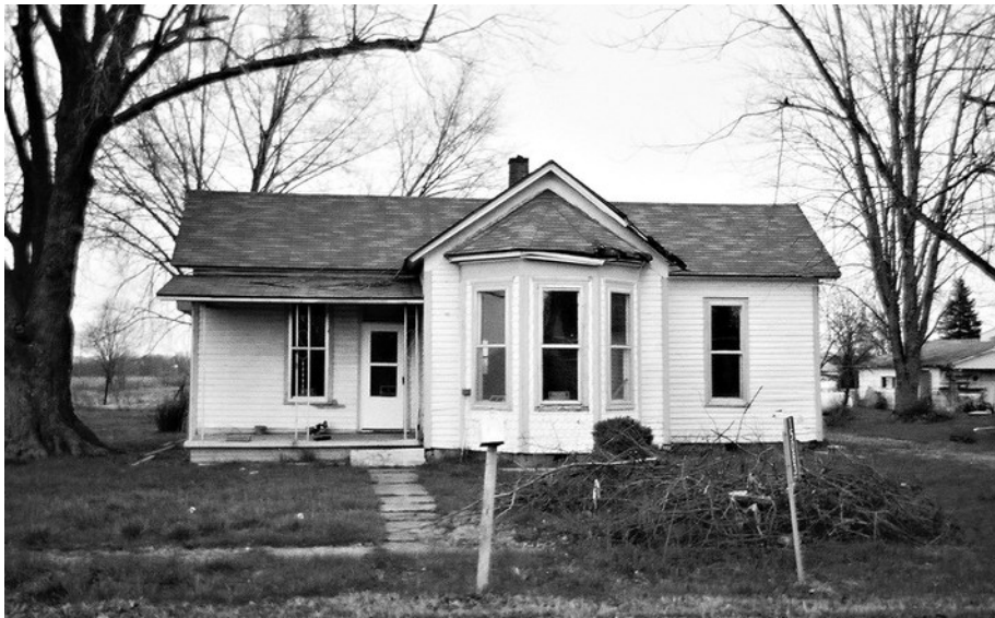
Lowther house in Oliver in 1995 (roof damage from recent storm)
